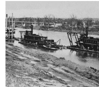
Two Corps snagboats and a dredge clear the Savannah River at Augusta, Ga., in the 1920s.
